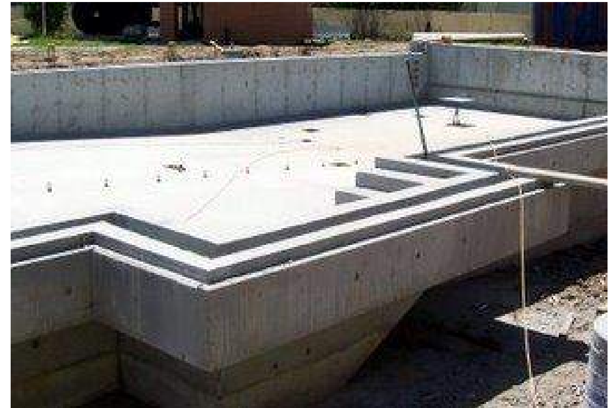
Figure 6.2: In-situ Reinforced Pool Tank Design at Grade
